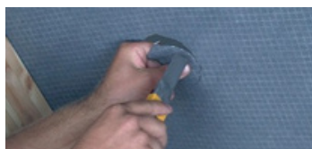
2 Once the location is confirmed, cut the hole in the underlay using a knife or jigsaw
