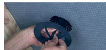
4 Feed the fixing strip through the centre of the lower section - the underlay should be between the lower section (inside) and the grill section (outside)
