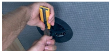
6 Cut off the excess of the fixing strip approx. 1cm above the lower section
