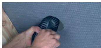
3 Holding firmly onto the fixing strip, squeeze the grill section of the KimaAir Inside-Out and push through the hole
