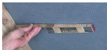
1 Mark out the location for a 111mm diameter hole on the underlay
