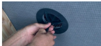
5 Press the lower section against the underlay and pull the fixing strip to tighten and lock the two sections together
